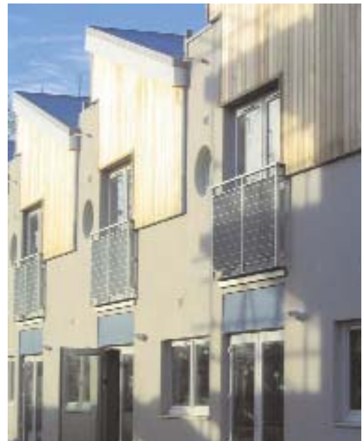
Western Challenge HA scheme: "86 new homes in Poole by Western Challenge Housing Association. EcoHomes 'very good' achieved at a cost of £84,884 per unit"
